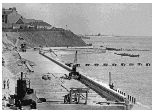
Pakefield Sea Wall under construction here in 1935
