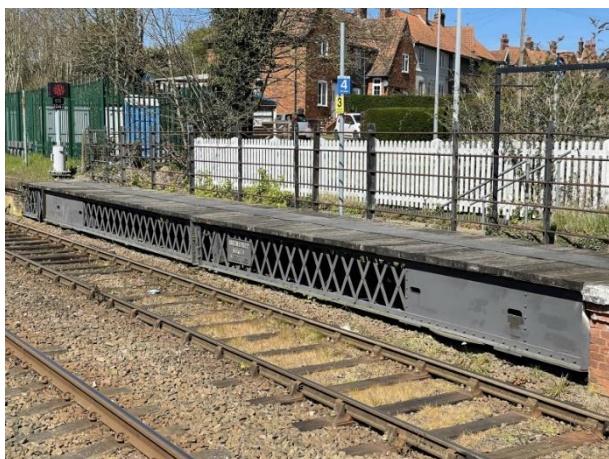
This picture shows the moveable platforms on one side of the railway lines.
